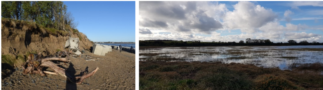
Sandy cliff erosion, Portrane beach, 09/2021 (left); Salt marshes of Rogerstown estuary (right). Photos by Iris Möller (TCD).
